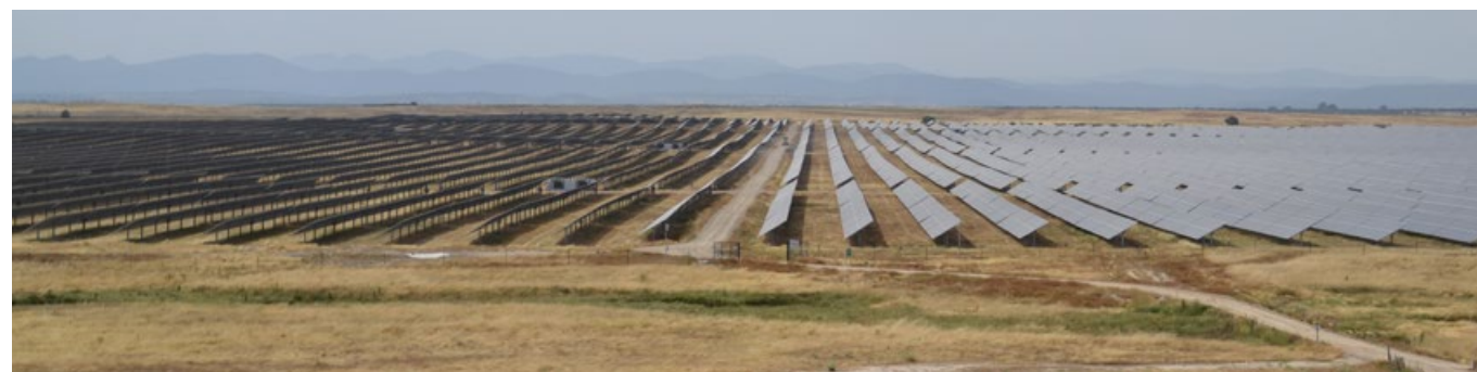
Solar plant in Spain, 300MW
