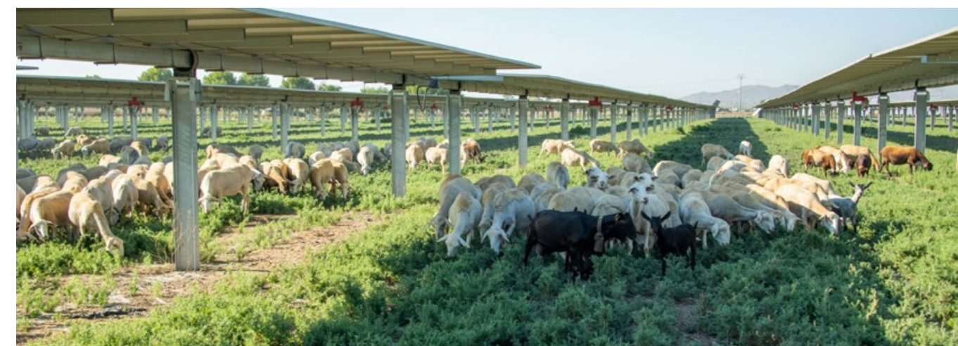
Solar plant in Spain, 85 MW.
