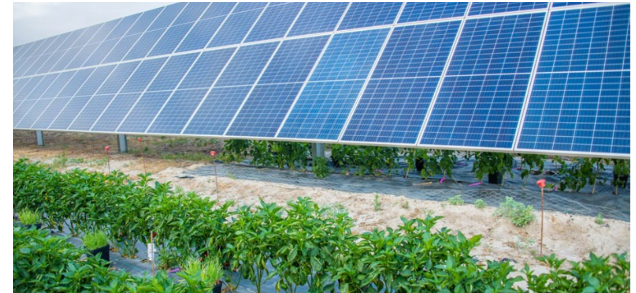
Solar plant in Spain, 85 MW.
