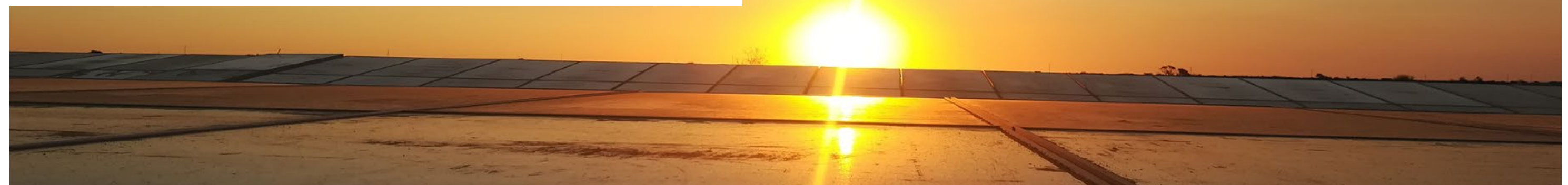
Solar plant in Namibia
